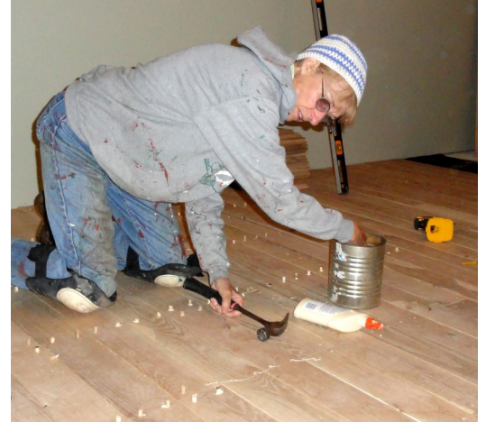
Linda Vance gluing in the hand made wooden plugs.
